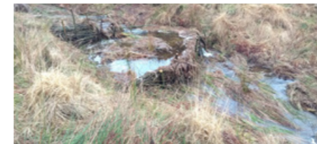
Willow faggot dam in a steep gully, Hoar Moor, Exmoor, February 2019. Willow was used in this situation to slow flows, trap sediments and create small areas of wet willow woodland. It was part of wider works to reinstate the River Quarme back into its original course, having been diverted in the early twentieth century.
