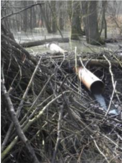
Figure 4-8. “Beaver Deceiver” flow device allows the height of the dam and extent of the flooding to be managed without destroying the dam or wetland (DWT 2016).
