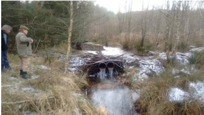
Figure 2-11. Example of a piped beaver dam in Scotland (photo courtesy of Dylan Roberts)
